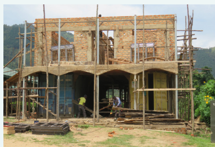
Containers being modified to office space
