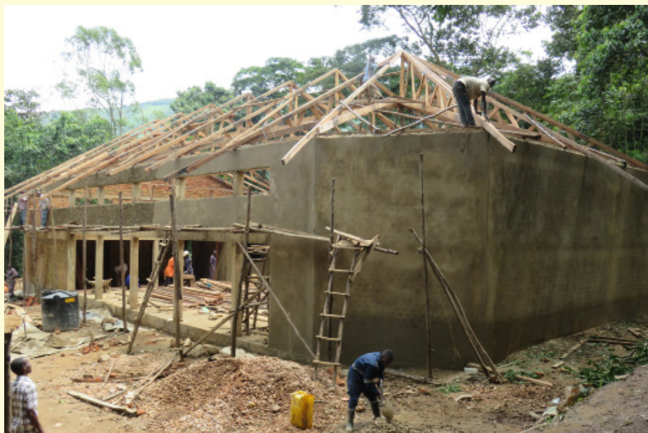
Multi- purpose banda under construction
